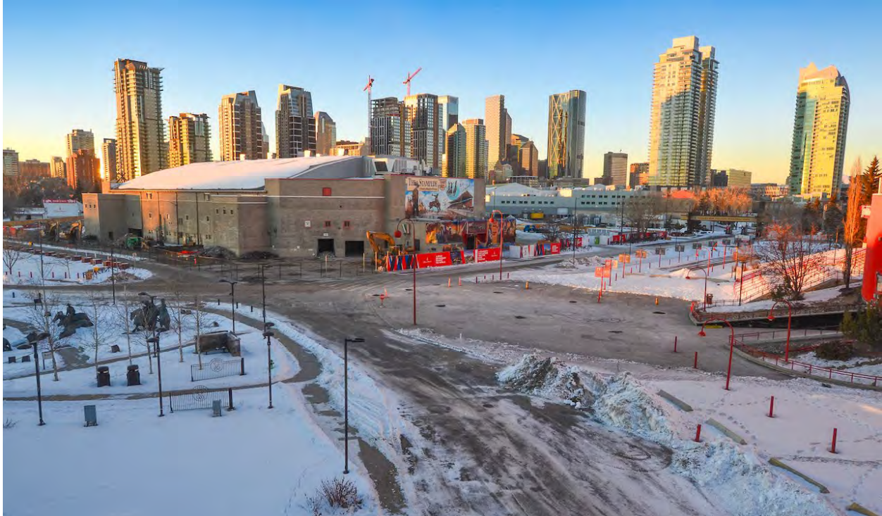
Looking northwest at Stampede Corral on the site of the future BMO Centre Expansion, image courtesy of CMLC and Calgary Stampede
