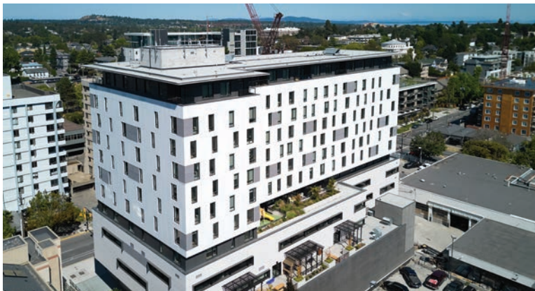
Eight storeys of affordable housing top the new Victoria Fire Station No. 1, which is designed to ensure immediate post-disaster occupancy.
