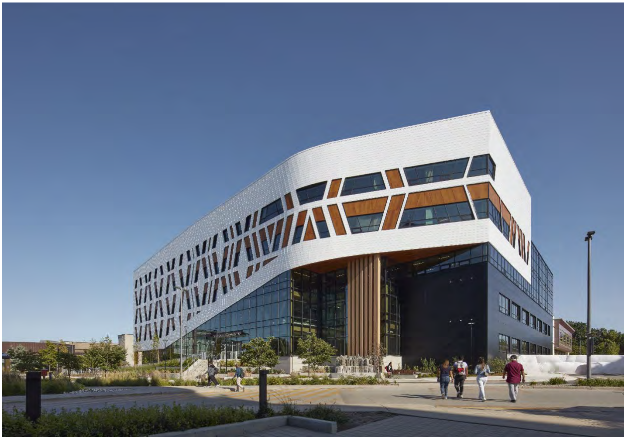
A-Building Expansion at Progress Campus, image courtesy of DIALOG
