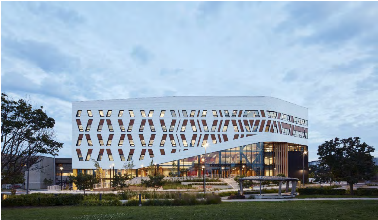
A-Building Expansion at Progress Campus, image courtesy of DIALOG
