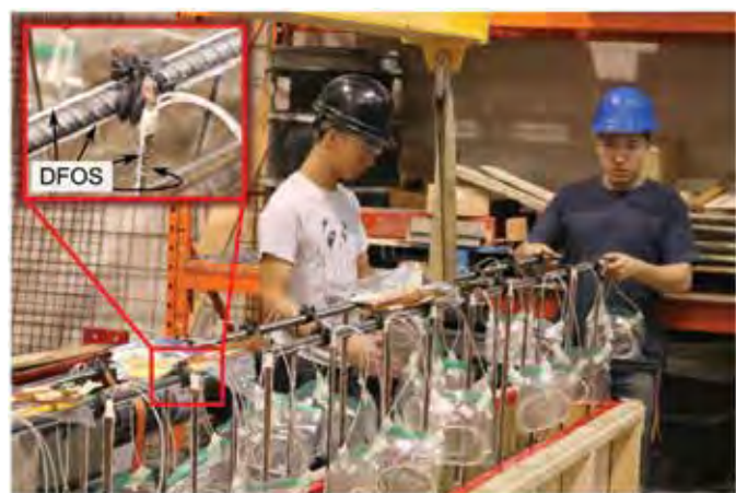
Fig. 3: Reinforcement cage of specimen JP-2 being lowered into the forms prior to concrete casting with DFOS bonded to the 20M reinforcement and 10M stirrups visible
