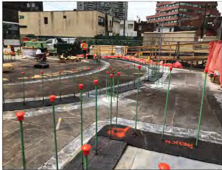
Ongoing installation of liquid-applied, hot rubberized waterproofing.
