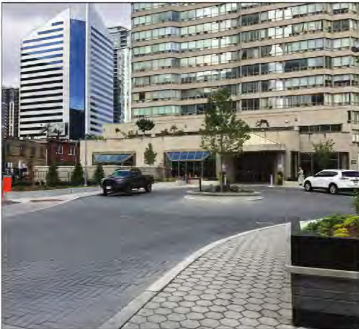
Completed podium restoration at 30 Greenfield Avenue.
