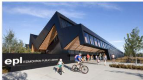
Capilano Library, Edmonton, Alta., designed by Patkau Architects Inc., is a 2020 recipient of the AIA/ALA Library Building Award by the American Institute of Architects (AIA) and the American Library Association (ALA). Photo courtesy James Dow + Patkau Architects
