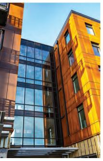
Lukas Farey, project manager, Campbell Construction Ltd., explains the cladding came with almost a stainless-steel look to it. "We applied a solution to the Corten that makes the oxidizing of the metal accelerate. Eventually the building would do that on its own over time." He adds the two buildings at Ironworks share a concrete podium, with a glazed walkway connecting the structures. "It acts as if it's one building, but during construction we built it as if it were two," he says
