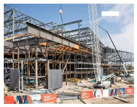
COURTESY CALGARY MUNICIPAL LAND CORPORATION — There are currently approximately 400 trade workers onsite, including steel, mechanical, electrical, drywall and concrete crews. In just 11 months, crews installed 9,000 metric tonnes of steel to form the structure
