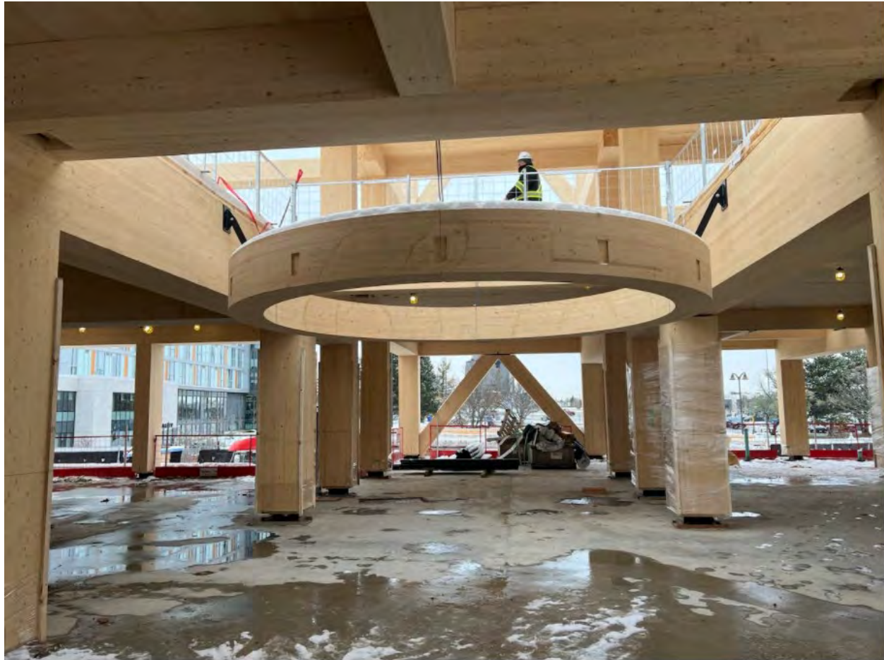
Centennial College Block A expansion, image provided by RJC Engineers
