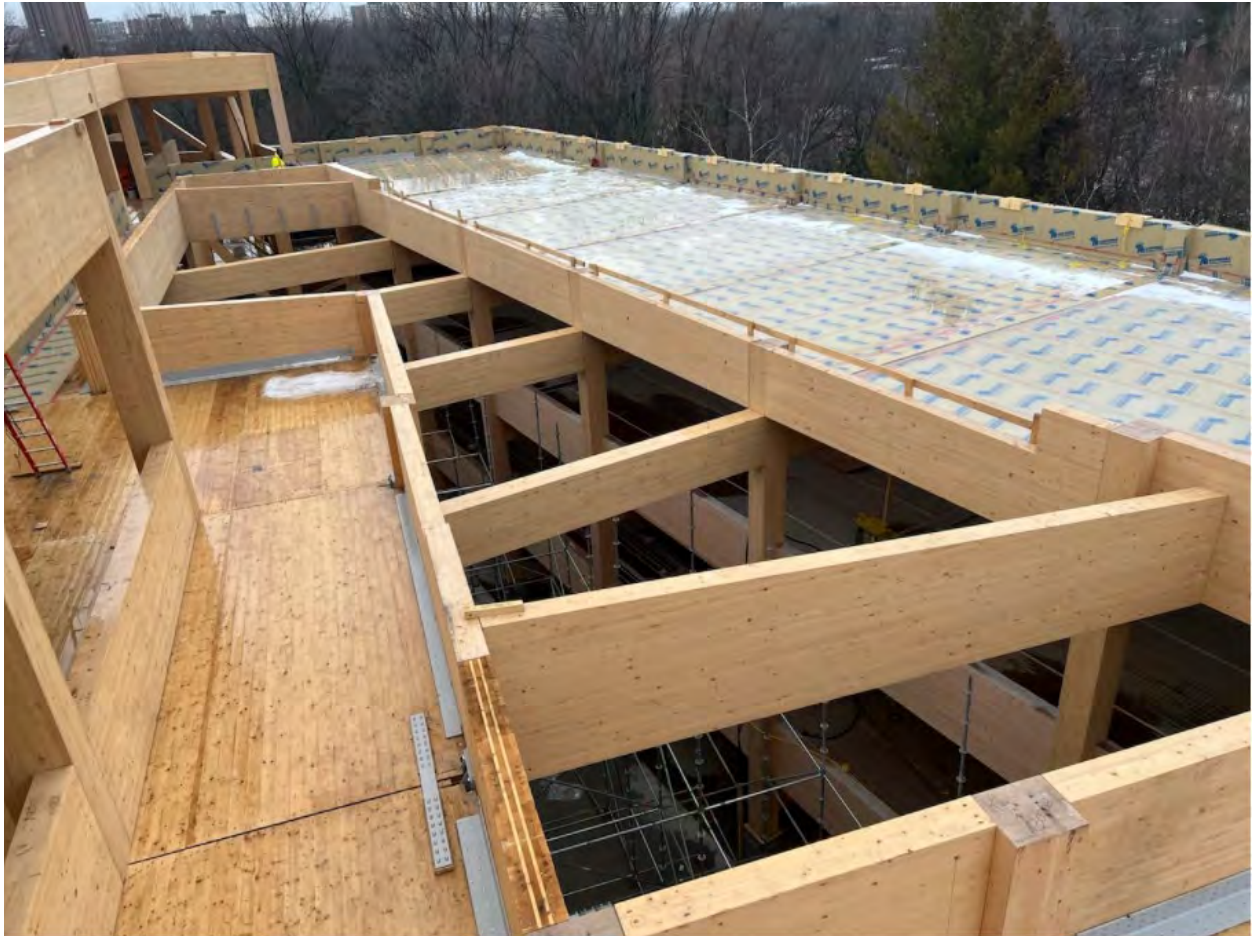
TRCA Administrative building, image provided by RJC Engineers
