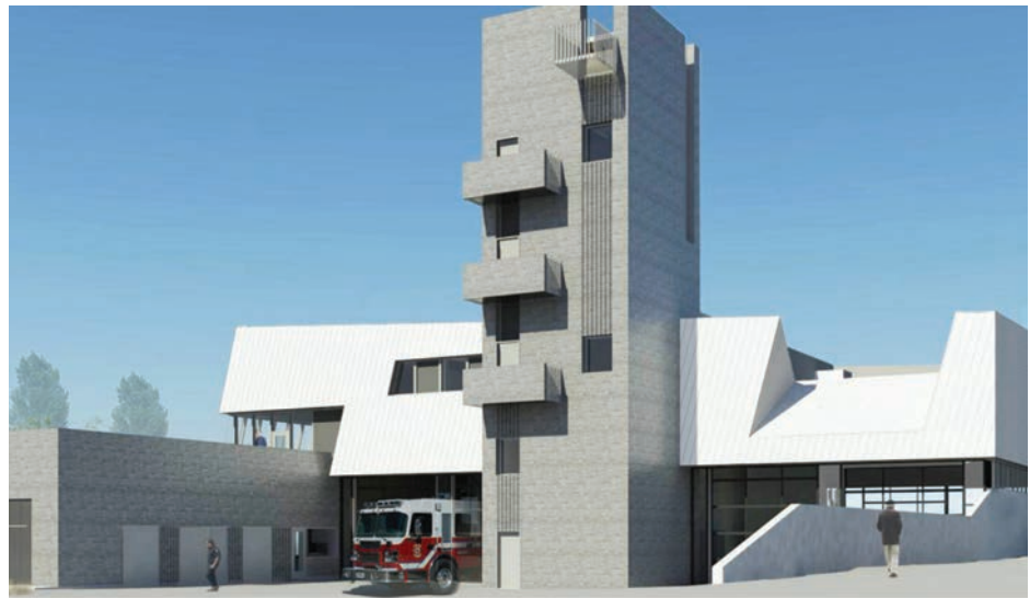
The fire hall has a sturdy concrete structure that serves as an armature for a steel frame on the upper levels where the exterior walls slope toward the central tower. The living and administration areas are thermally isolated from the apparatus bay below and the six-storey training tower with a variety of structural thermal breaks.
