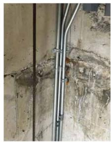
Water stains on the foundation wall are an indication that leakage has occurred and an inspection should be conducted to assess where it's coming from and how to prevent it. Any signs of water in an elevator pit have the potential for trouble.
