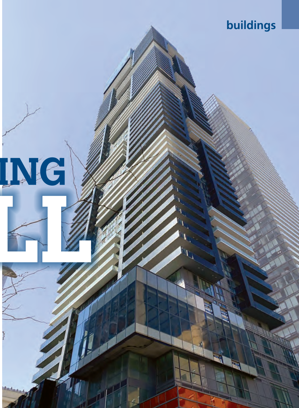
The 63-story YC Condos building is a tall slender building with a world's first damping system.
