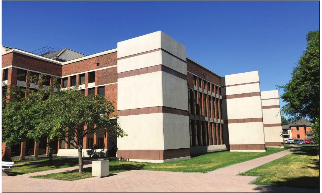
Overview of typical shear walls with granite panel recesses.
