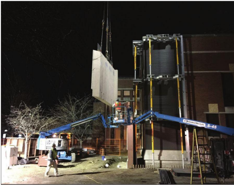
Shear wall installation during construction.
