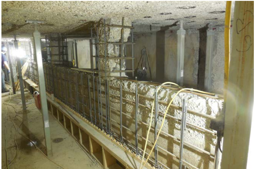
Overlay reinforcement on the Influent Channel No. 2's overflow weir.
