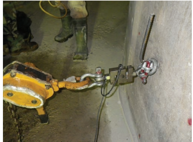
Fig. 16: Load testing of dowels
