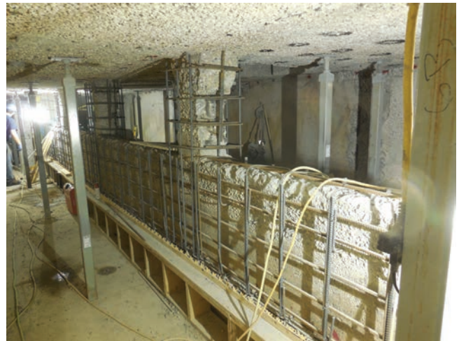
Fig. 9: Formwork, bracing and drilling of reinforcing dowels
