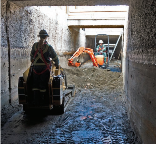
Fig. 5: Initial removal of channel debris
