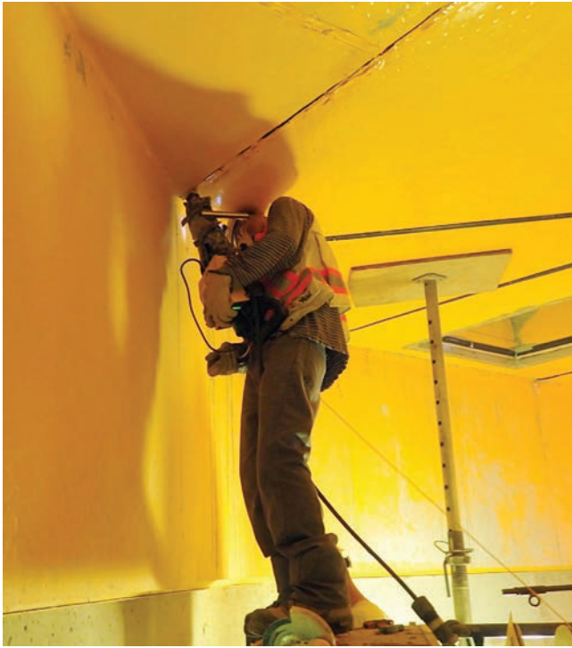
Fig. 14: Field welding of HDPE liner seams
