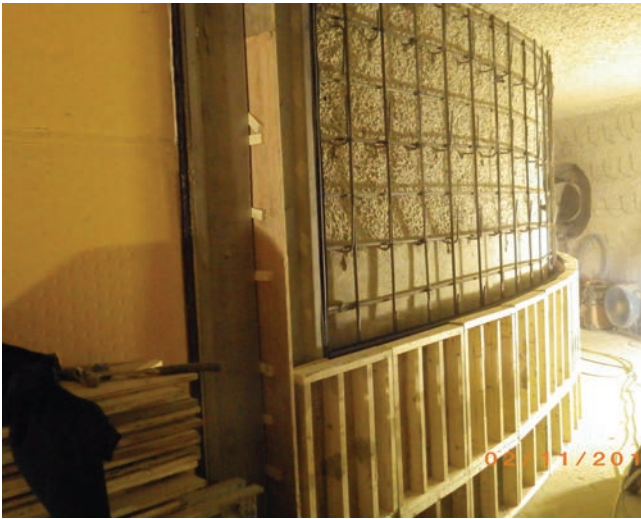
Fig. 11: Wall liner, reinforcement, and formwork
