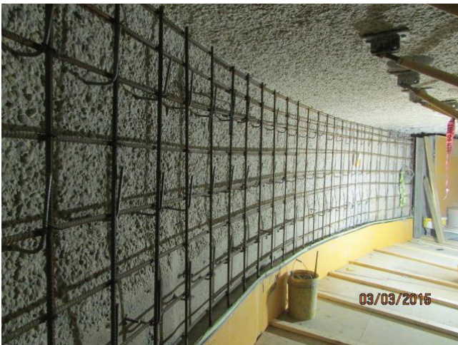
Fig. 7: Reinforcing and base of HDPE liner at curved wall
