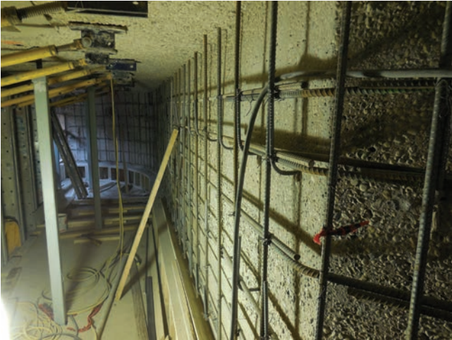
Fig. 6: Wall reinforcing and bracing
