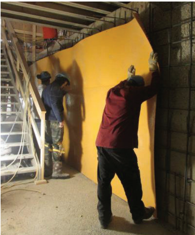
Fig. 13: Trial fit of HDPE liner prior to erection of formwork
