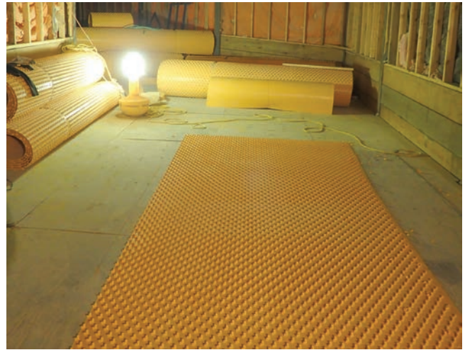
Fig. 8: Preparation of HDPE liner for installation
