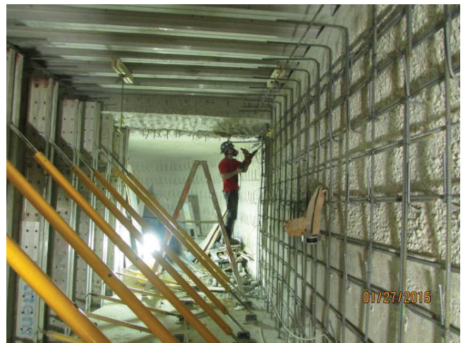
Fig. 10: Overlay reinforcement at overflow wier
