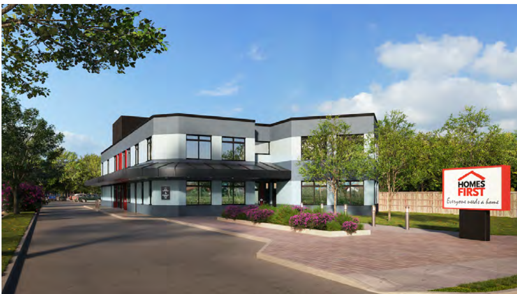
4117 Lawrence Avenue from the front, image courtesy of RJC Engineers
