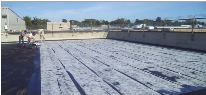
Installation of first ply and reinforcing for hot-rubberized waterproofing system.
